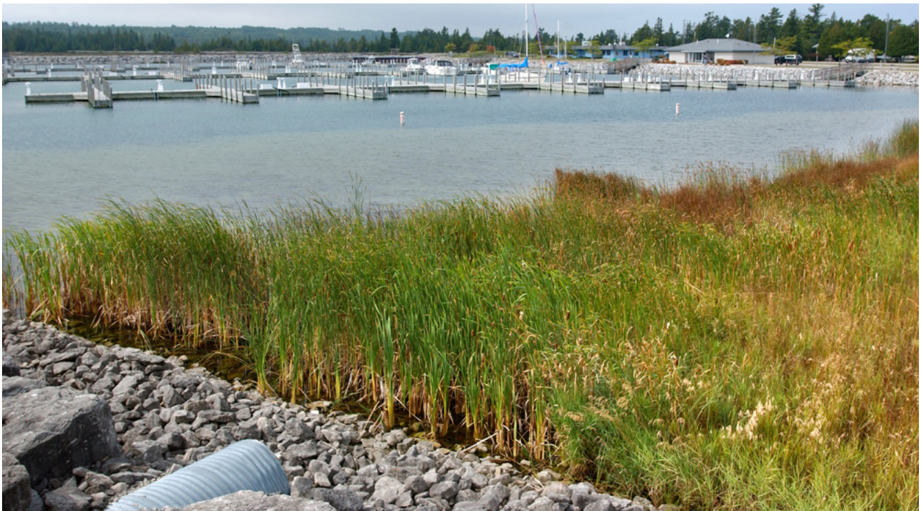
Bioswales: An example of an environmental mitigation measure that can be included in marinas and special waterfront provisions. (Todd Marsee, Michigan Sea Grant)
